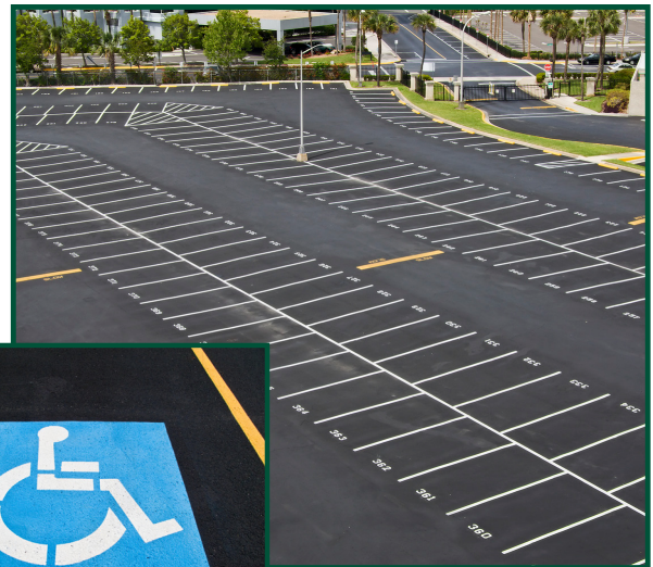
Parking Lot Striping
